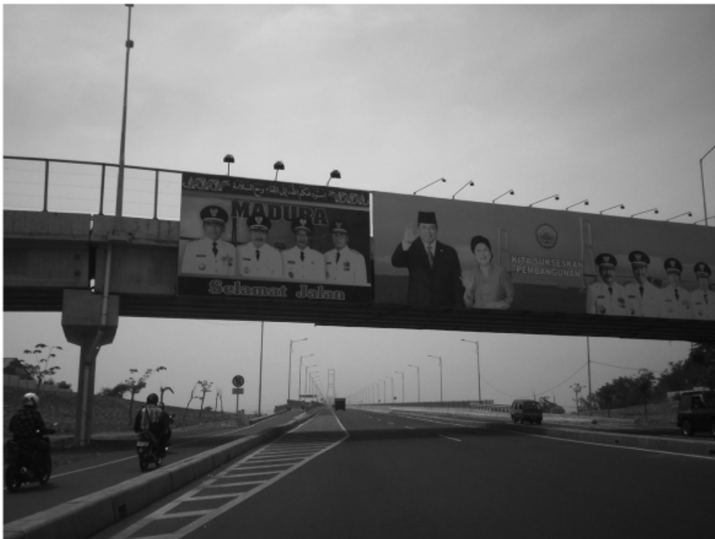
Figure 5.1 The Suramadu Bridge seen from the Madura side
